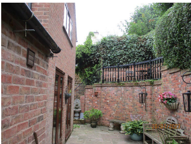
Rear elevation, garden and boundary wall.
